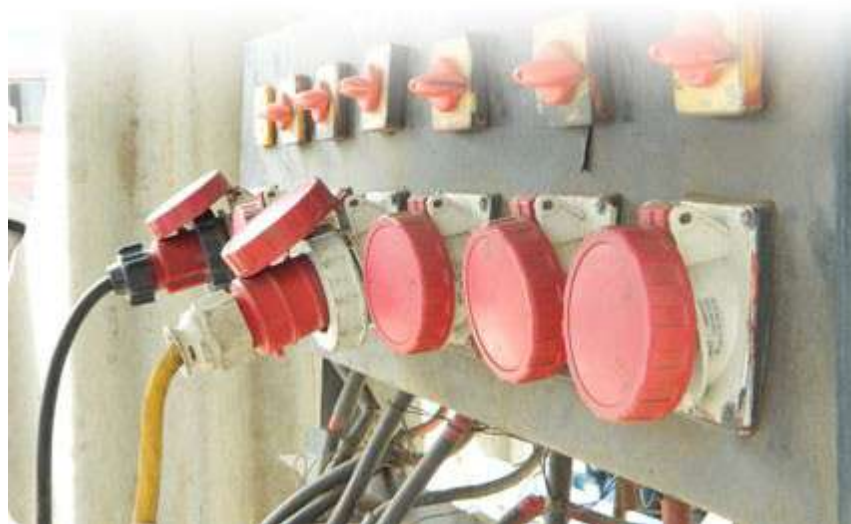
440V switchboard used by Ship's crew for plugging / unplugging Reefers
